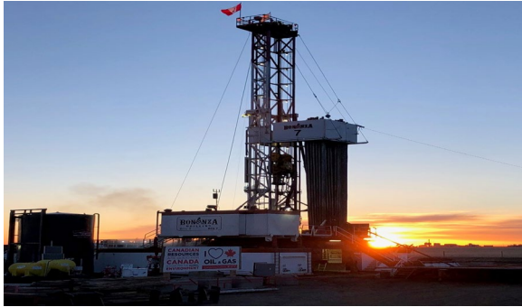
Drilling an open hole Sunburst well in Brooks
