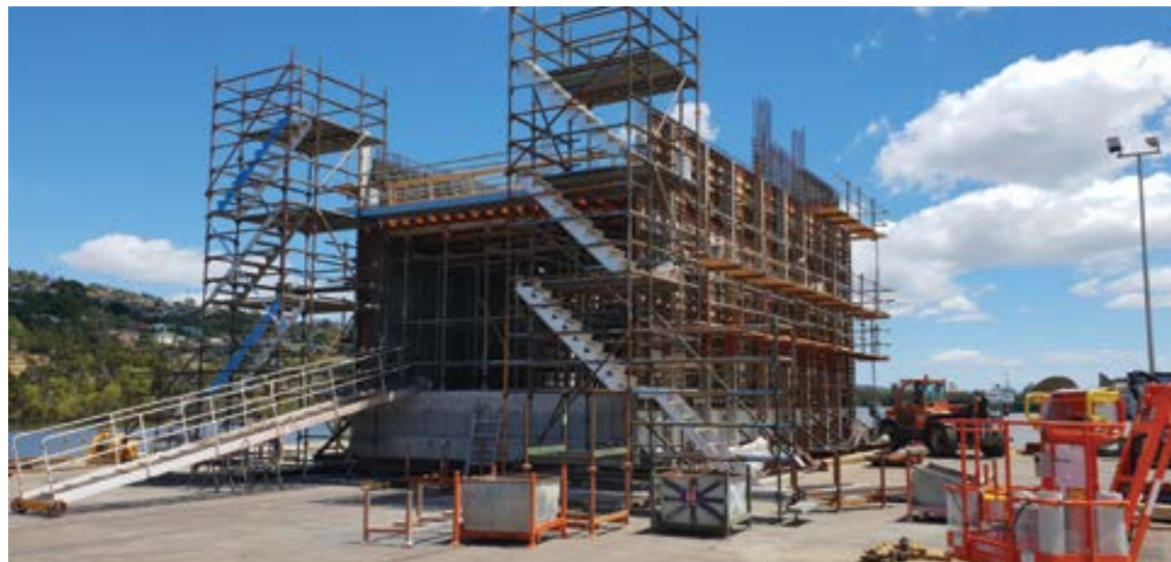
Below: King Island OWC under construction
